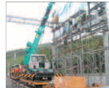
Construction in progress
