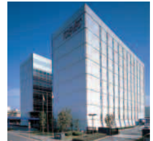
Head Office Annex
