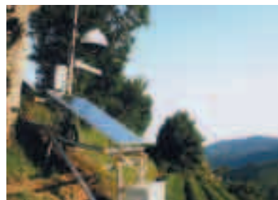
Landslide monitor camera
