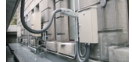
▲Seismic isolation of external cable
