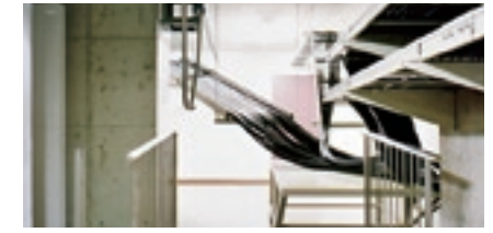
▲Communication cable of extra length for seismic isolation displacement
