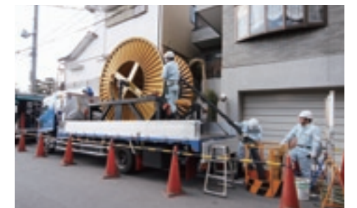
Underground cable construction
