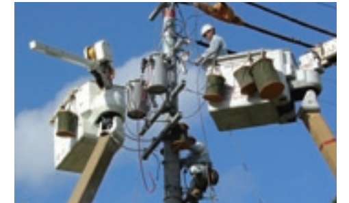
Electric wiring construction
