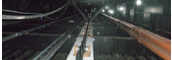
▲Inside the bridge superstructure
