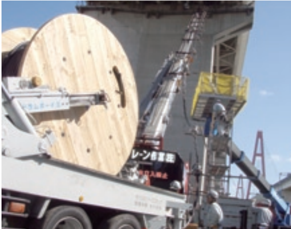
▲New cable being installed
