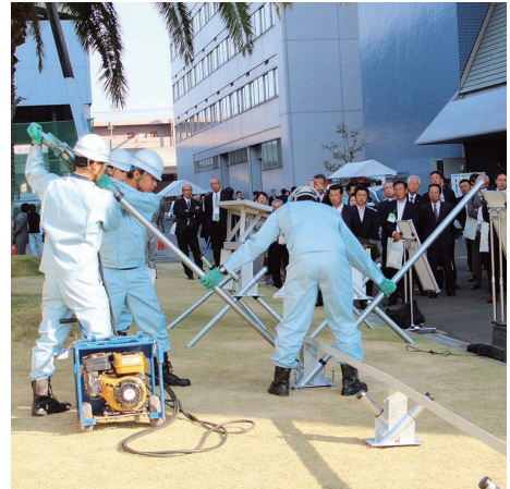
▲Demonstration of assembly work for FX Steel Pipe Stand
