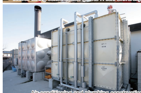
Air-conditioning and plumbing construction
