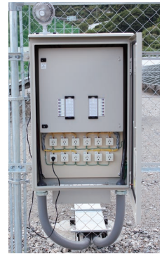
▲Emergency power supply unit
