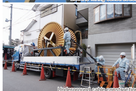
Electric wiring construction
