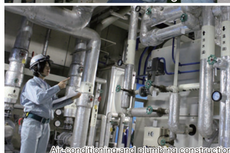
Air-conditioning and plumbing construction
