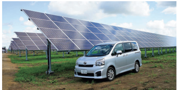
▲Panels were installed at higher positions in preparation for accumulated snowfall, and the solar altitude was also taken into consideration.
