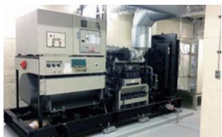
▲Emergency power generator
