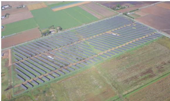
▲Panels were installed at higher positions in preparation for accumulated snowfall, and the solar altitude was also taken into consideration.
