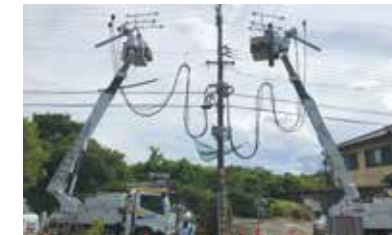
Work using the indirect live wire work method
