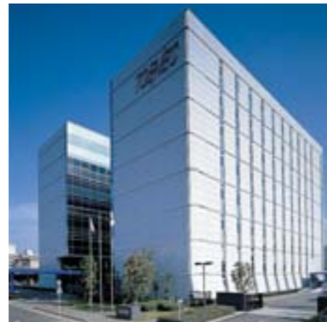
Head Office Annex
