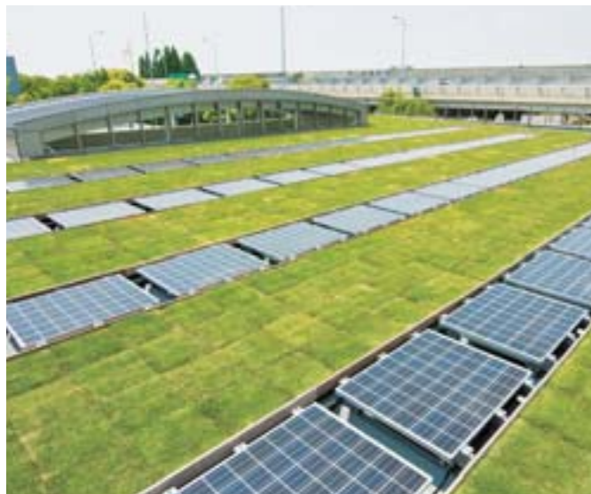
The rooftop at the visitor center comprise solar panels and grass belts.
