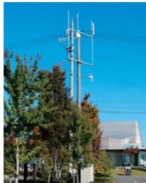
A WiMAX station
