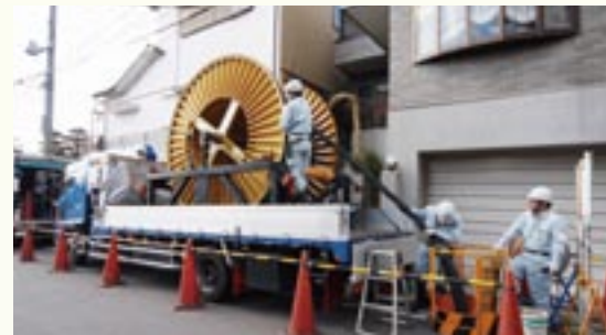
Underground cable construction
