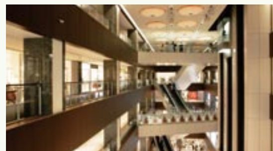
Indoor-wiring construction (photo : Midland Square)
