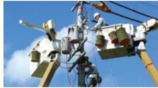
Electric wiring construction
