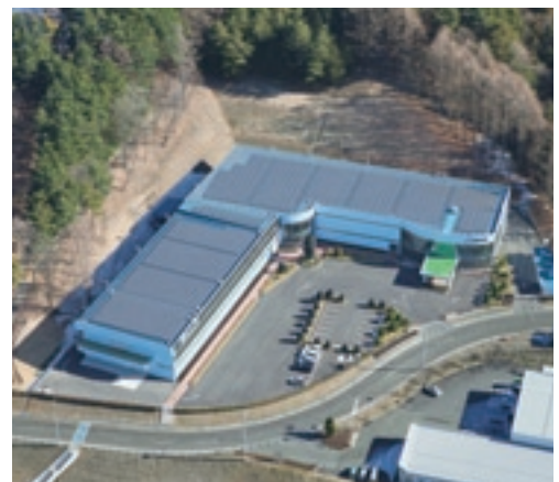
▲Solar panels installed on rooftop
