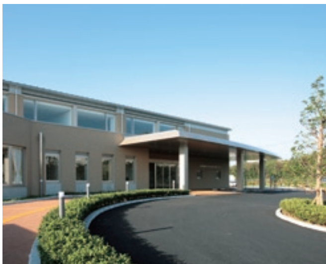
▲Western Community Center
