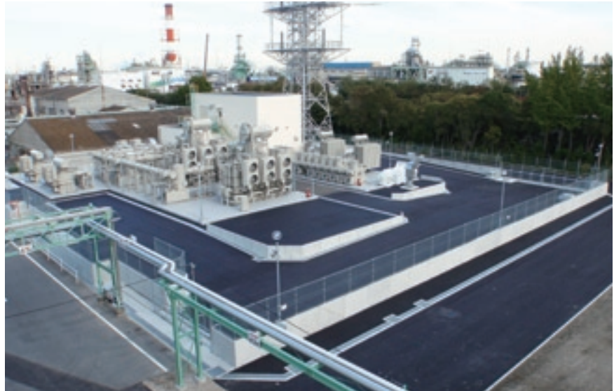
▲High Voltage Substation, Chiba Plant, Asahi Glass Co., Ltd.
