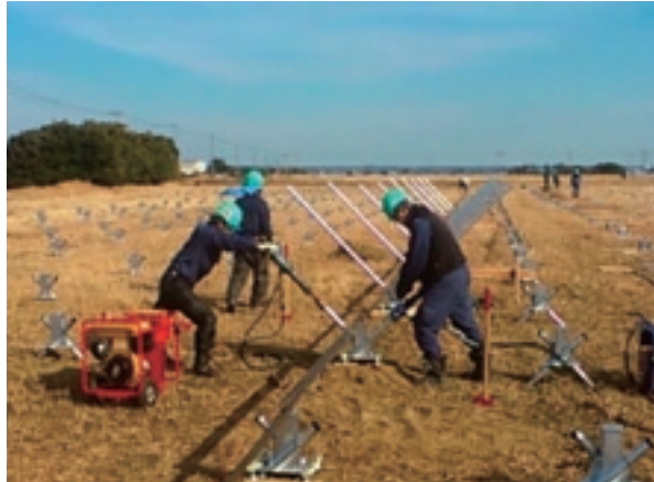
▲Workers installing the FX Steel Pipe Stand
