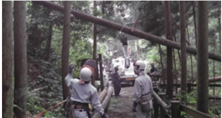
▲Restoration work in Shizuoka Prefecture
