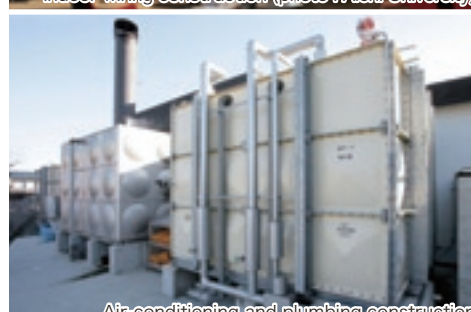
Air-conditioning and plumbing construction
