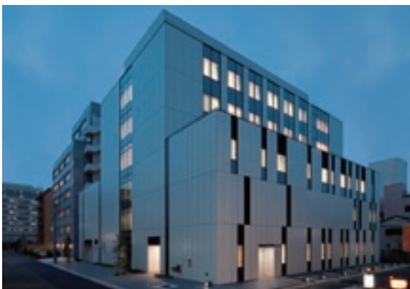
▲South Wing of the Kamiida Daiichi General Hospital
