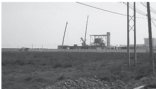
▲ Planned location for the substation
