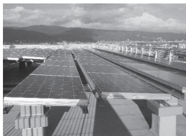
▲Rooftop photovoltaic facilities
