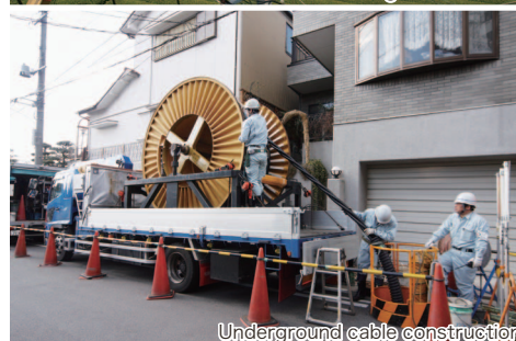
Underground cable construction
