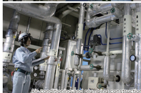
Air-conditioning and plumbing construction
