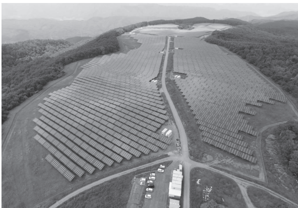
▲ Solar panels installed to match the undulating terrain
