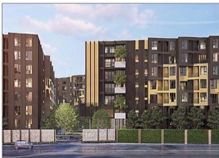
Project : The Base Central Phuket Owner : Sansiri Area : 28,000 M 2 Room : 590 Units Scope : M&E System Contract : Direct / Sansiri Amount : 111 MB
