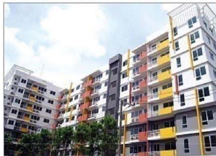
Project : My Condo SKV 52 Owner : Sansiri Area : 8,000 M 2 Room : 146 Units Scope : EE System Contract : Direct / VP Amount : 10 MB
