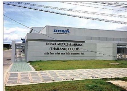
Project : DMM Project Location : Amata City Estate (Rayong) System : Electrical, A/C & Ventilation, Sanitary & Pumping Fire Fighting Building Area : 4,300 SQM Capacity of Transformer : 1,880 KVA Term : 2012
