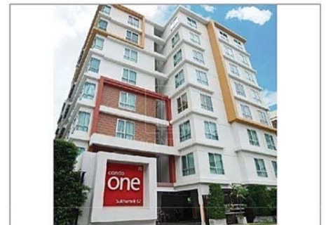
Project : Condo One SKV 67 Owner : Plus Property Area : 8,000 M 2 Room : 80 Units Scope : EE System Contract : Indirect / VP Amount : 7 MB
