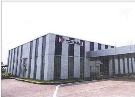
Project : Yokohama Rubber Location : Hemarht Industrial Estate System : Electrical, A/C & Vantilation, Sanitary & Pumping, Fire Fighting Building Area : 2,200 SQM Capacity of Transformer : 680 KVA Term : 2008
