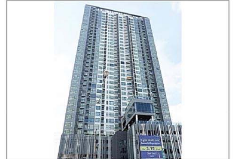
Project : Rhythm Asoke I Owner : AP Area : 25,000 M 2 Room : 385 Units Scope : M&E System Contract : Direct / AP Amount : 120.5 MB
