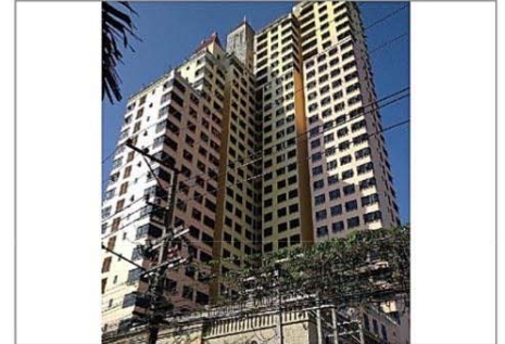
Project : The Crest Phahol 11 Owner : SC Asset Area : 19,000 M 2 Room : 154 Units Scope : M&E System Contract : Direct / SC Asset Amount : 65 MB
