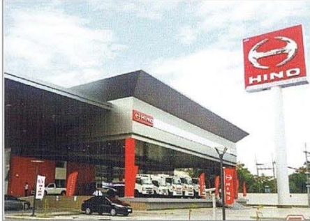
Project : Hino Showroom Location : Leamchabang Chonburi System : Electrical System Building Area : 7,000 SQM Capacity of Transformer : 500 KVA Term : 2015
