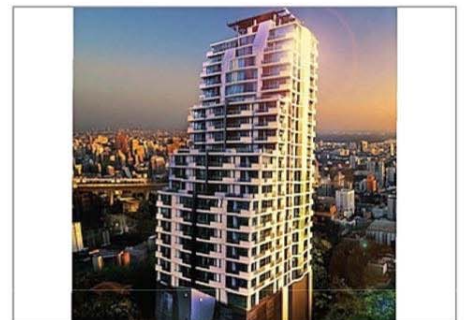
Project : Le Monaco Owner : French Company Area : 30,000 M 2 Room : 68 Units Scope : M&E System Contract : Indirect / Pre-built Amount : 107 MB
