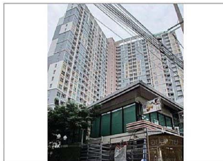
Project : Rich Park Condo Bangson Owner : Richy Area : 39,800 M 2 Room : 802 Units Scope : M&E System Contract : Indirect / TTS Amount : 130 MB
