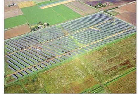
Project : Toenec Eniwa Solar Power Plant Purpose : Solar Power Plant Completion : 2014 Area : Hokkaido Numbers of Panel : 18,600 Capacity : 4,000 KW
