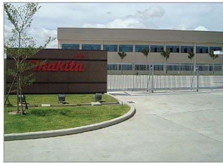
Project : Makita Location : Phinthon 3 (Chonburi) System : Electrical, A/C & Vantilation, Sanitary & Pumping, Process & Utility, Fire Fighting Buiding Area : 32,000 SQM Capacity of Transformer : 4,500 KVA Term : 2011
