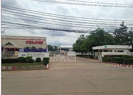
Project : Thai GMB Industrial Location : 304 Industrial Estate System : Electrical, A/C & Vantilation, Sanity & Pumping Process & Utility, Fire Fighting Buiding Area : 14,000 SQM Capacity of Transformer : 4,000 KVA Term : 2010
