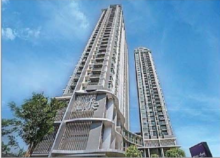
Project : Life Ratchada Owner : AP Area : 70,000 M 2 Room : 837 Units Scope : M&E System Contract : Direct / VP Amount : 260 MB
