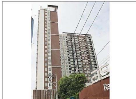
Project : Aspire Rattana Thibase II Owner : AP Area : 83,000 M 2 Room : 1,428 Units Scope : M&E System Contract : Direct / AP Amount : 324 MB
