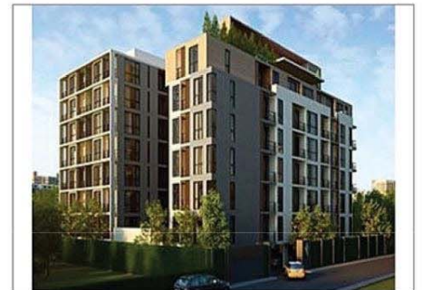
Project : The Base SKV 50 Owner : Sansiri Area : 24,000 M 2 Room : 415 Units Scope : M&E System Contract : Indirect / TTS Amount : 89 MB
