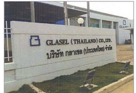
Project : Glasel (Thailand) Location : Bang Phrian, Bang Bo, Samutprakan System : Electrical A/C & Clean room Buiding Area : 6,700 SQM Capacity of Transformer : 2,250 KVA Term : 2014
