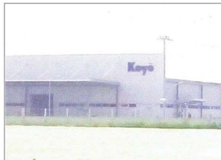
Project : Koyo Joint Location : Bangpho Industrial Estate System : Electrical & Process Utility Building Area : 5,800 SQM Capacity of Transformer : 3,000 KVA Term : 2015
