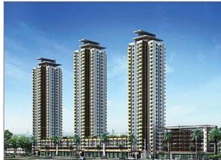
Project : M-Society Condo Owner : MTR Area : 65,000 M 2 Room : 1,046 Units Scope : M&E System Contract : Direct / MTR Amount : 190 MB
