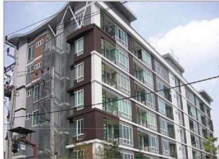
Project : The Muse Owner : Dpec Area : 8,000 M 2 Room : 80 Units Scope : M&E System Contract : Direct Amount : 23.5 MB
