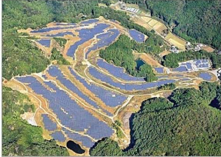
Project : Tochigi West Solar Power Plant Purpose : Solar Power Plant Completion : 2019 Area : Tochigi Prefecture
