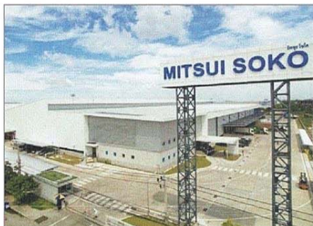
Project : Mitsui Soko Location : Bangna-Trad Rd, KM19 System : Electrical System Building Area : 18,000 SQM Capacity of Transformer : 1,000 KVA Term : 2013
