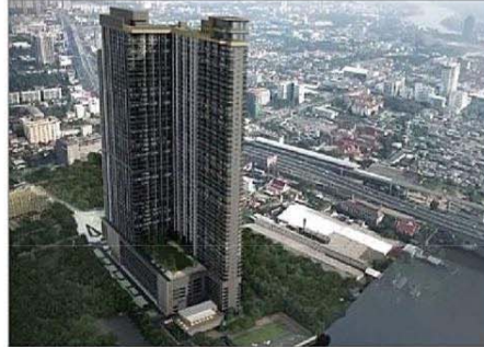
Project : The Politan Rive Phase I Owner : Everland Area : 152,700 M 2 Room : 2,300 Units Scope : M&E System Contract : Direct / Everland Amount : 490 MB
