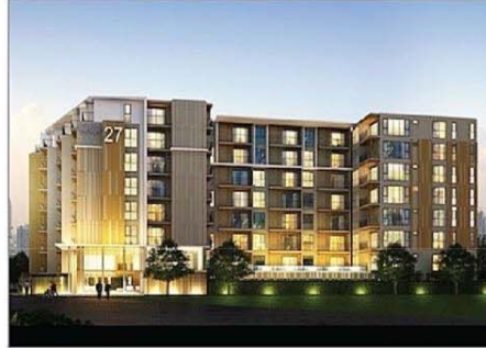
Project : Mirage SKV 27 Owner : Mirage Area : 15,000 M 2 Room : 117 Units Scope : M&E System Contract : Direct Amount : 43 MB
