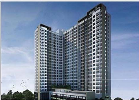
Project : Aspire Sathorn Ratchapreuk Owner : AP Area : 65,000 M 2 Room : 1,087 Units Scope : M&E System Contract : Indirect / SMC Amount : 190 MB
