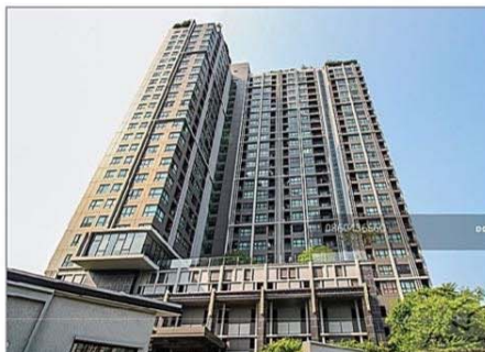
Project : The Line SKV 71 Owner : Sansiri Area : 23,000 M 2 Room : 313 Units Scope : EE&AC System Contract : Indirect / TTS Amount : 53.5 MB
