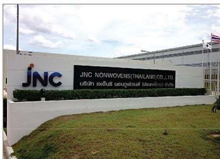
Project : JNC Project Location : Amata City Estate (Rayong) System : A/C & Ventilation, Sanitary & Pumping Process & Utility, Fire Fighting Building Area : 8,000 SQM Capacity of Transformer : N/A Term : 2012
