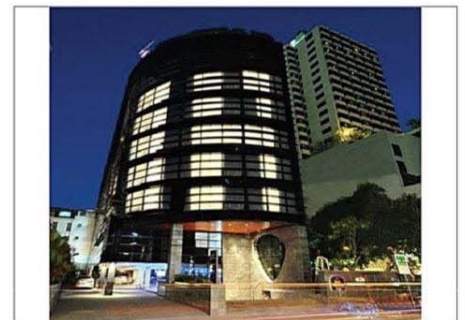
Project : BW@20 Owner : The Tropical Area : 10,000 M 2 Room : 78 Units Scope : M&E System Contract : Direct / The Tropical Amount : 53 MB
