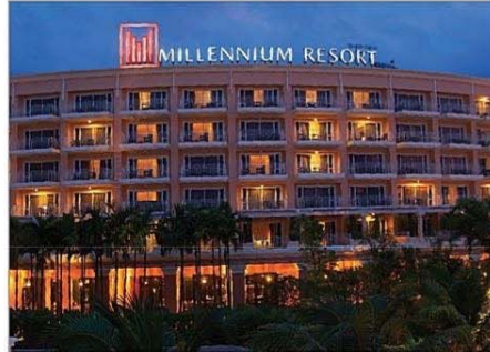
Project : Millennium Beach Side Patong Owner : MTR Area : 20,000 M 2 Room : 197 Units Scope : M&E System Contract : Direct / MTR Amount : 150 MB
