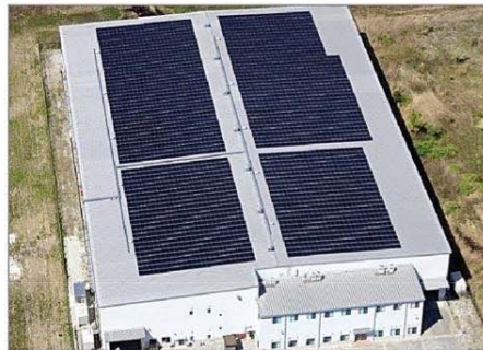
Project : U-NETRANS Tawara Distribution Center Purpose : Distribution Center Completion : 2014 Area : Aichi Prefecture Numbers of Panel : 3,048 Capacity : 500 KW
