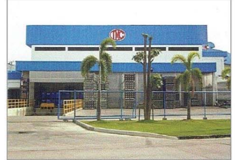
Project : TMC PA Factory Location : Saha Rattana Nakhorn Industrial Estate System : Electrical, A/C & Vantilation, Sanitary & Pumping, Fire Fighting Building Area : 2,100 SQM Capacity of Transformer : 1,000 KVA Term : 2008
