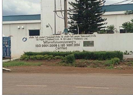
Project : Oji Label Location : 304 Industrial Estate System : Electrical, A/C & Vantilation, Sanity & Pumping Buiding Area : 4,200 SQM Capacity of Transformer : N/A Term : 2010
