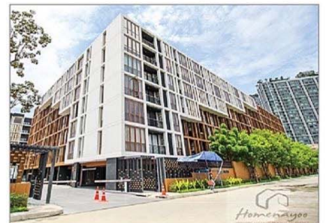
Project : Hasu Huas Owner : Sansiri Area : 20,000 M 2 Room : 333 Units Scope : M&E System Contract : Indirect / TTS Amount : 81.3 MB
