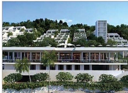
Project : The Naihan Owner : MTR Area : 5,000 M 2 Room : 130 Units Scope : M&E System Contract : Direct / MTR Amount : 158 MB
