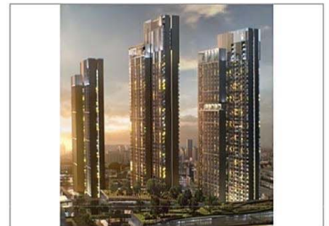
Project : Whizdom Inspire Sukhumvit 101 (R) Owner : MQDC Area : 55,000 M 2 Room : 554 Units Scope : M&E System Contract : Direct / MQDC Amount : 300 MB
