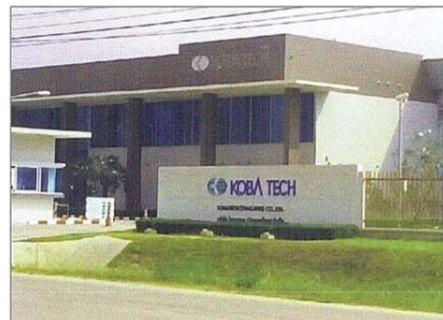
Project : Kobatech Location : Banbung Chonburi System : Electrical Building Area : 11,000 SQM Capacity of Transformer : 4,500 KVA Term : 2013
