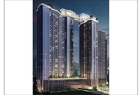
Project : Life Asoke-RAMA IV Owner : AP Area : 150,000 M 2 Room : 2,248 Units Scope : M&E System Contract : Direct / AP Amount : 410 MB
