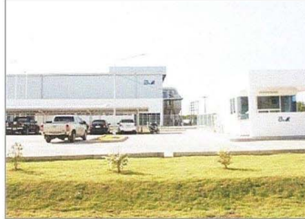
Project : A&M Casting Location : Rachaburi IE Rachaburi System : Electrical Building Area : 5,200 SQM Capacity of Transformer : 2,630 KVA Term : 2015
