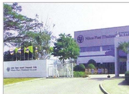
Project : Nihon Plast Location : Amata City Industrial Estate System : Electrical Building Area : 5,200 SQM Capacity of Transformer : 2,000 KVA Term : 2014
