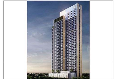
Project : Whizdom Connect SKV 101 Owner : MQDC Area : 42,200 M 2 Room : 673 Units Scope : M&E System Contract : Direct / MQDC Amount : 188.8 MB
