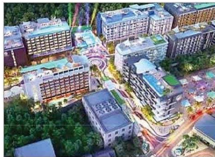
Project : The Beach Plaza Phase I Owner : K.W. Plaza Area : 13,683 M 2 Room : 291 Units Scope : M&E System Contract : Direct / K.W. Plaza Amount : 143 MB
