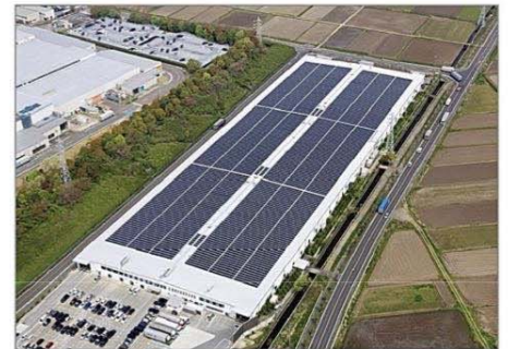
Project : U-NETRANS Miyoshi Distribution Center Purpose : Distribution Center Completion : 2014 Area : Aichi Prefecture Numbers of Panel : 10,872 Capacity : 1,800 KW
