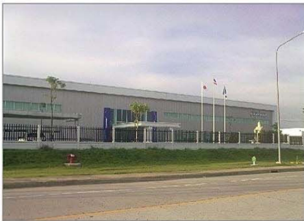
Project : Clarion Location : Eastern Seaboard System : Electrical, Clean Room Buiding Area : 11,000 SQM Capacity of Transformer : 3,315 KVA Term : 2011
