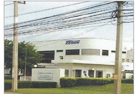
Project : Keihin New Warehouse Location : Rojana Ayuthaya Industrial Estate System : Electrical, A/C & Vantilation, Sanitary & Pumping, Fire Fighting Building Area : 1,250 SQM Capacity of Transformer : NA Term : 2010
