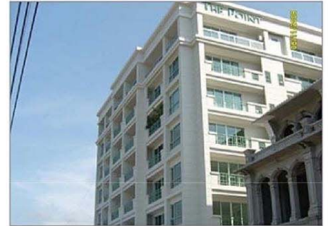
Project : The Point Owner : Local Company Area : 8,000 M 2 Room : 80 Units Scope : M&E System Contract : Direct Amount : 18.5 MB
