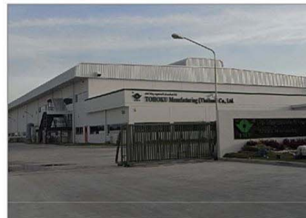
Project : Tohoku Location : Phinthon 1 (Chonburi) System : Electrical, A/C & Vantilation, Sanitary & Pumping, Process & Utility, Fire Fighting Buiding Area : 6,000 SQM Capacity of Transformer : 3,000 KVA Term : 2012
