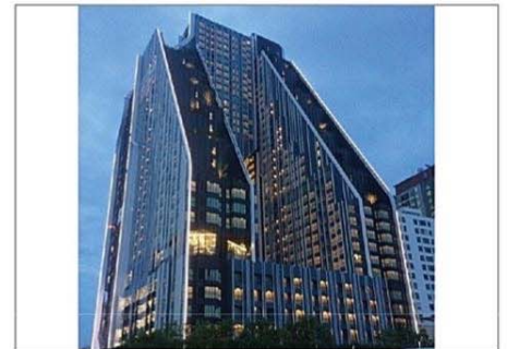
Project : Ideo-Q Chula-Samyam Owner : Ananda Area : 97,500 M 2 Room : 1,598 Units Scope : EE System Contract : Indirect / VP Amount : 155.1 MB
