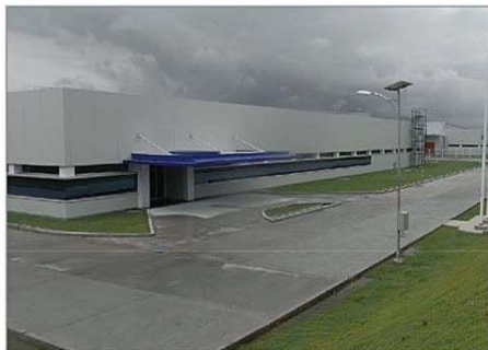
Project : NMT Project Location : Phinthong Industrial Estate (Phinthong 3 Chonburi Province) System : Electrical, A/C & Ventilation, Sanitary & Pumping, Process & Utility, Fire Fighting Building Area : 14,000 SQM Capacity of Transformer : 4,000 KVA Term : 2012
