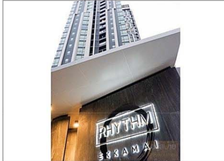
Project : Rhythm Eakkamai Owner : AP Area : 28,500 M 2 Room : 326 Units Scope : M&E System Contract : Direct / AP Amount : 99.5 MB
