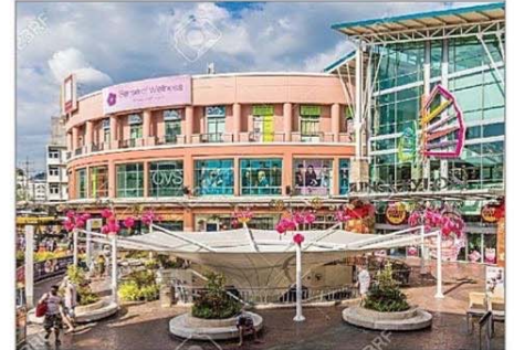
Project : Jungceylon Phuket Owner : MTR Area : 25,000 M 2 Scope : M&E System Contract : Direct / MTR Amount : 150 MB
