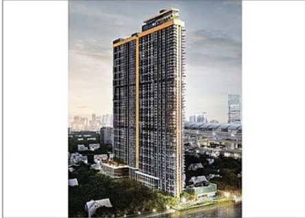
Project : The Politan Aqua Owner : Everland Area : 170,000 M 2 Room : 2,751 Units Scope : M&E System Contract : Direct / Everland Amount : 505 MB
