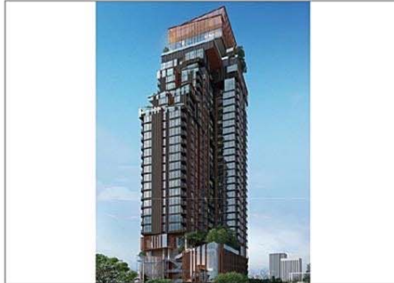
Project : Rhythm Eakkamai Estate Owner : AP Area : 33,000 M 2 Room : 203 Units Scope : M&E System Contract : Direct / AP Amount : 125 MB
