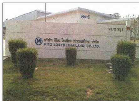
Project : Mito Kogyo Location : Pinthong 1 IE Chonburi System : Electrical Building Area : 5,400 SQM Capacity of Transformer : 400 KVA Term : 2014
