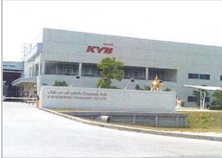
Project : KYB Sterling Location : Amata Nakorn Industrial Estate System : Electrical, A/C & Vantilation, Sanitary & Pumping, Fire Fighting Buiding Area : 18,000 SQM Capacity of Transformer : 2,500 KVA Term : 2012
