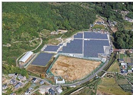
Project : Toenec Kumano Solar Power Plant Purpose : Solar Power Plant Completion : 2013 Area : Mie Prefecture Numbers of Panel : 9,912 Capacity : 19,990 KW
