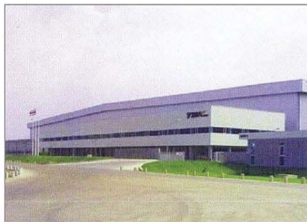
Project : TBKK Location : Amata Nakorn Industrial Estate System : Electrical Building Area : 37,000 SQM Capacity of Transformer : 6,000 KVA Term : 2015
