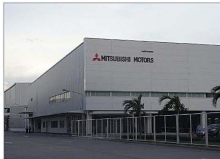
Project : MMTH (Misubishi Motr) Location : Leamchabang Estate System : Electrical, A/C & Ventilation, Sanitary & Pumping, Process & Utility, Fire Fighting Building Area : 18,000 SQM Capacity of Transformer : 4,500 KVA Term : 2012
