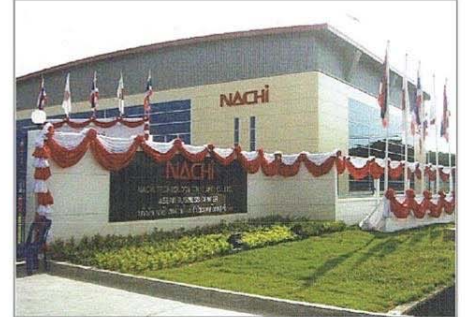
Project : Nachi Head Quarter Location : Rojana Rayong Industrial Estate System : Electrical, A/C & Vantilation, Sanitary & Pumping, Process & Utility, Fire Fighting Buiding Area : 2,400 SQM Capacity of Transformer : 500 KVA Term : 2008
