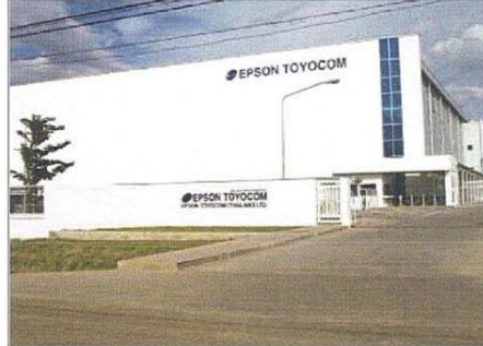
Project : Epson Toyocom Location : Gateway Industrial Estate System : Electrical A/C & Clean Room Buiding Area : 20,000 SQM Capacity of Transformer : 7,500 KVA Term : 2008
