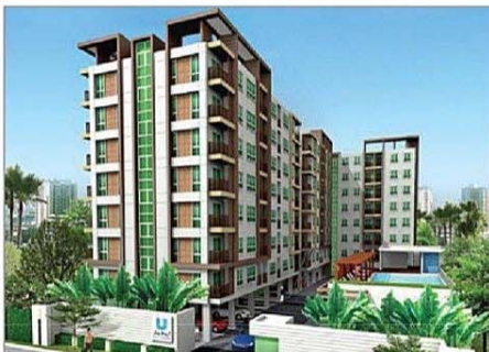
Project : U-Sabai Owner : Grand U Area : 8,000 M 2 Room : 139 Units Scope : M&E System Contract : Indirect / AP Amount : 14 MB
