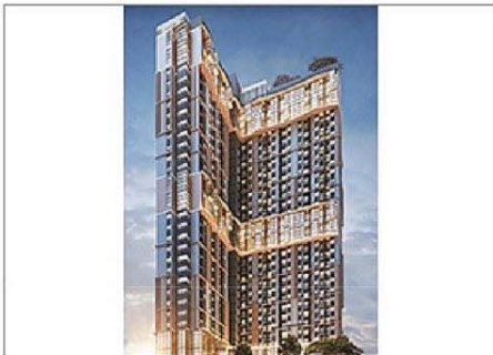
Project : Life Sathorn Sierra Owner : AP Area : 131,000 M 2 Room : 1,971 Units Scope : M&E System Contract : Direct / AP Amount : 406 MB
