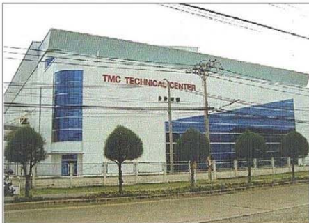
Project : TMC TECHNICAL CENTER Location : SAHA RATTANA NAHHORN INDUSTRIAL ESTASTE System : ELECTRICAL A/C & VENTILATION, SANITARY & PUMPING, FIRE FIGHTING Buiding Area : 5,000 SQM Capacity of Transformer : 2,000 KVA Term : 2008
