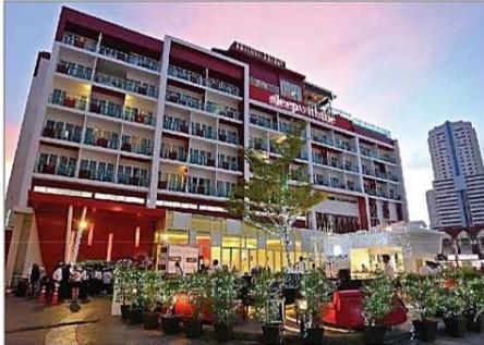
Project : Sleep With Me Hotel Owner : SWM Area : 23,000 M 2 Room : 258 Units Scope : M&E System Contract : Direct Amount : 154 MB
